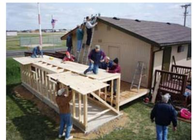
The next phase was attachment of the external sheathing which went fairly quickly. Before the day was done, members hoisted all the roof trusses up on to the building.
